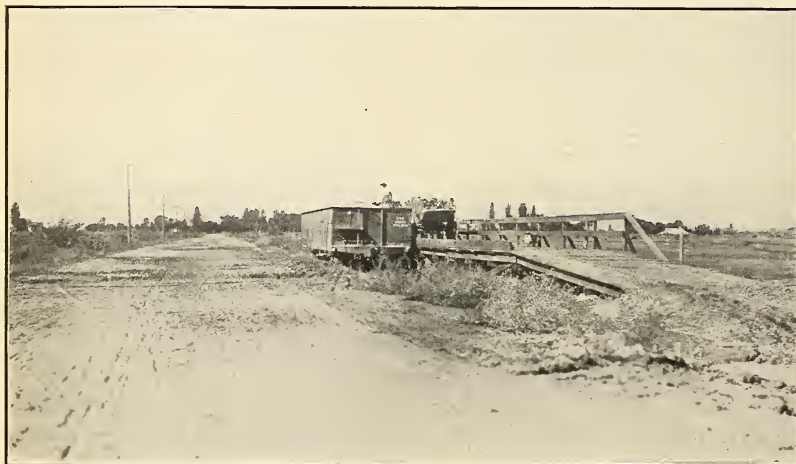
FIG. 2.—A POOR TYPE OF LOADING STATION. THE BEETS MUST BE LOADED IN RAILROAD CAR WITH FORKS.
